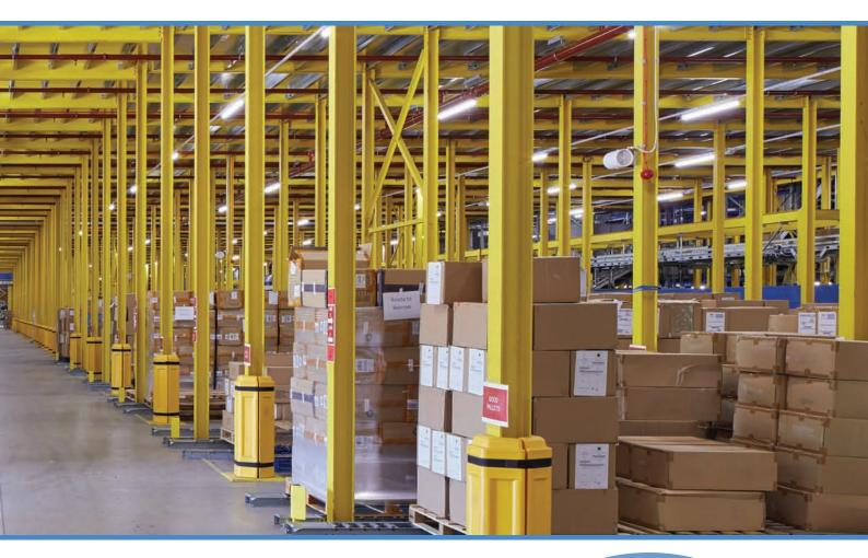
To avoid compromising on floor space, they devised a design to minimise the amount of visible upright steel columns used to support the new mezzanine.
